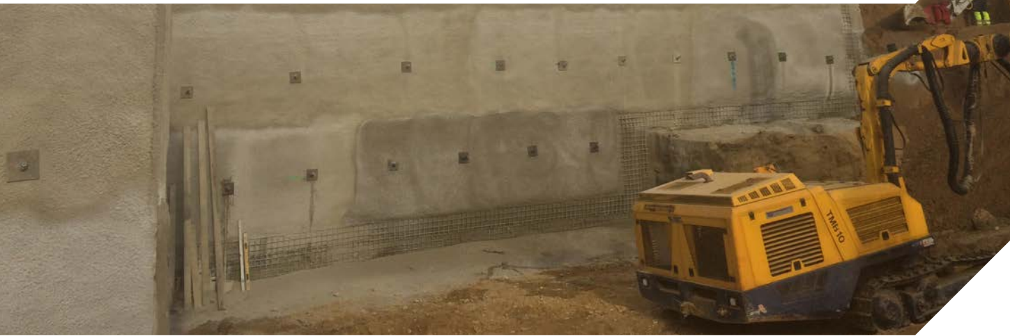
Soil nail with hollow bar
