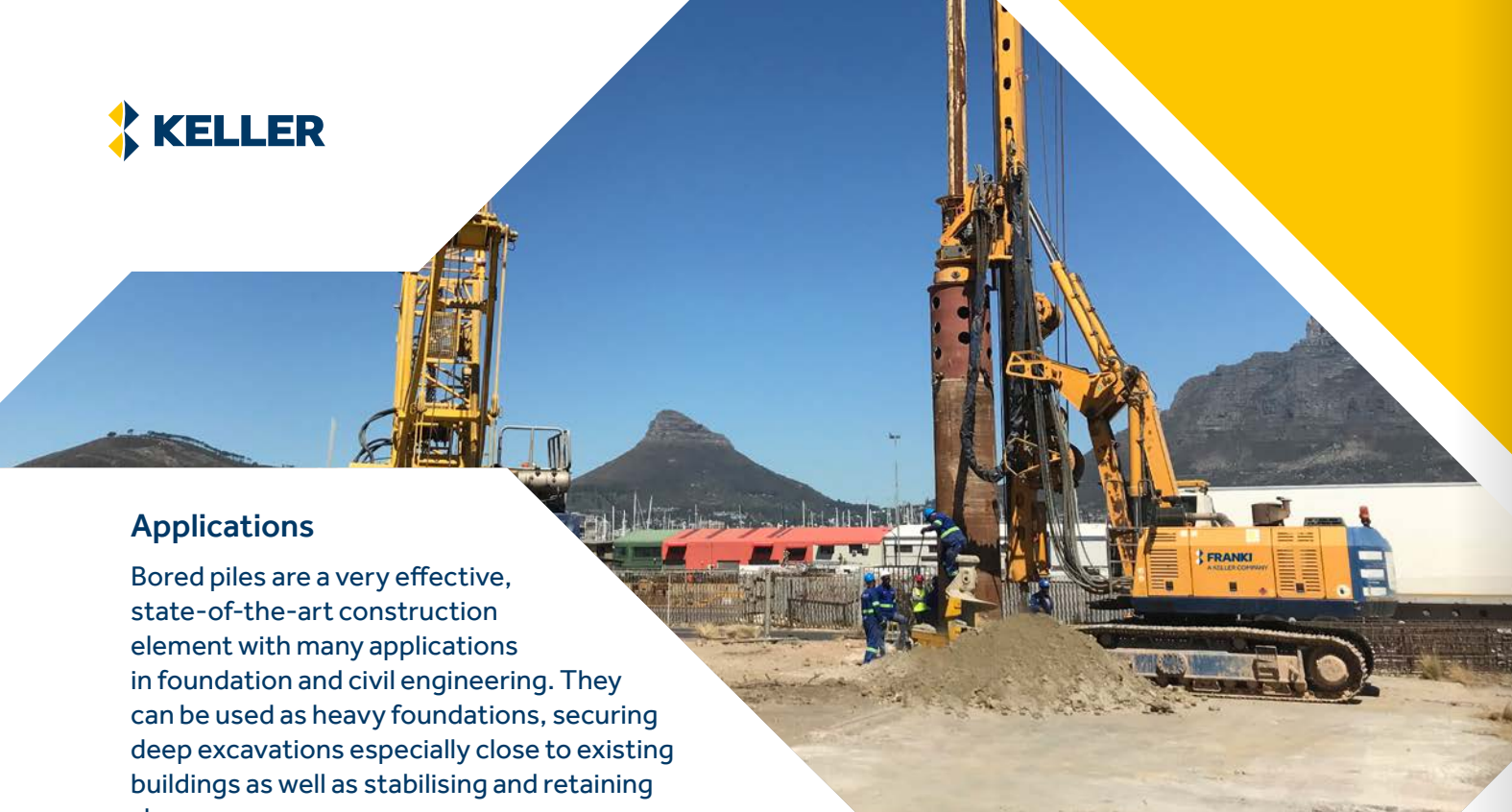
Casing installation and concreting
